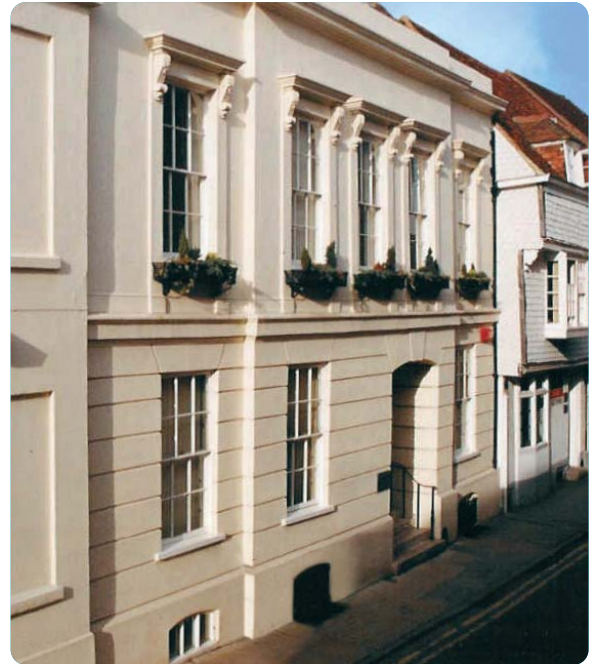
CLT main building in Castle Street
